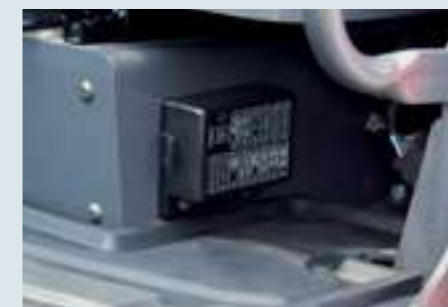
Convenient Fuse Box
