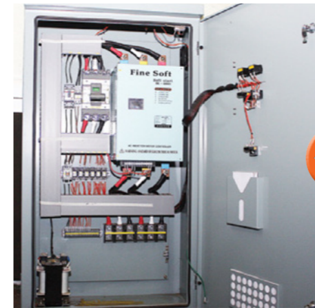
Control panel For main power supply
